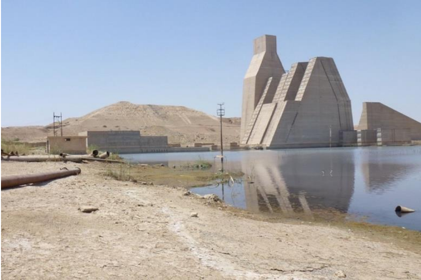
Figure 4. The Badush Dam abandoned construction site
