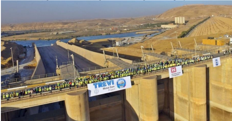
Figure 5. Trevi's engineers working at MD's project
